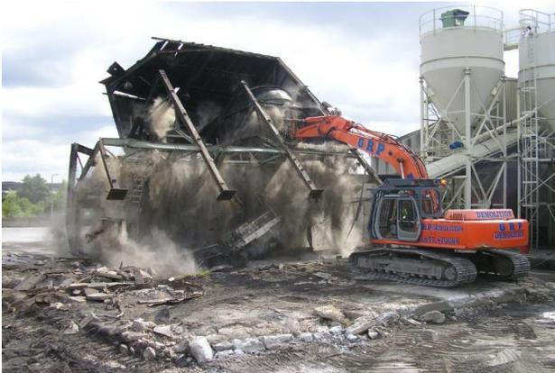
GRP dismantled portal frame buildings for resale and demolished a variety of structures including concrete ovens and a 30 meter steel chimney. The project was completed in a 12 week duration
