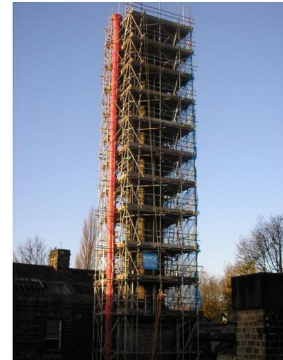
GRP completed the hand demolition of a 100ft chimney and subsidiary buildings using mechanical excavators at the former Springfield Works Mill, Guiseley for Chartford Homes. Restrictions were enforced due to live railway line which ran adjacent to the site and surrounding residential buildings.
