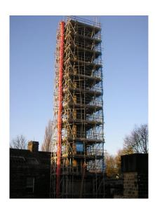
GRP completed the hand demolition of a 100ft chimney and subsidiary buildings using mechanical excavators at the former Springfield Works Mill, Guiseley for Chartford Homes.Restrictions were enforced due to live railway line which ran adjacent to the site and surrounding residential buildings.
